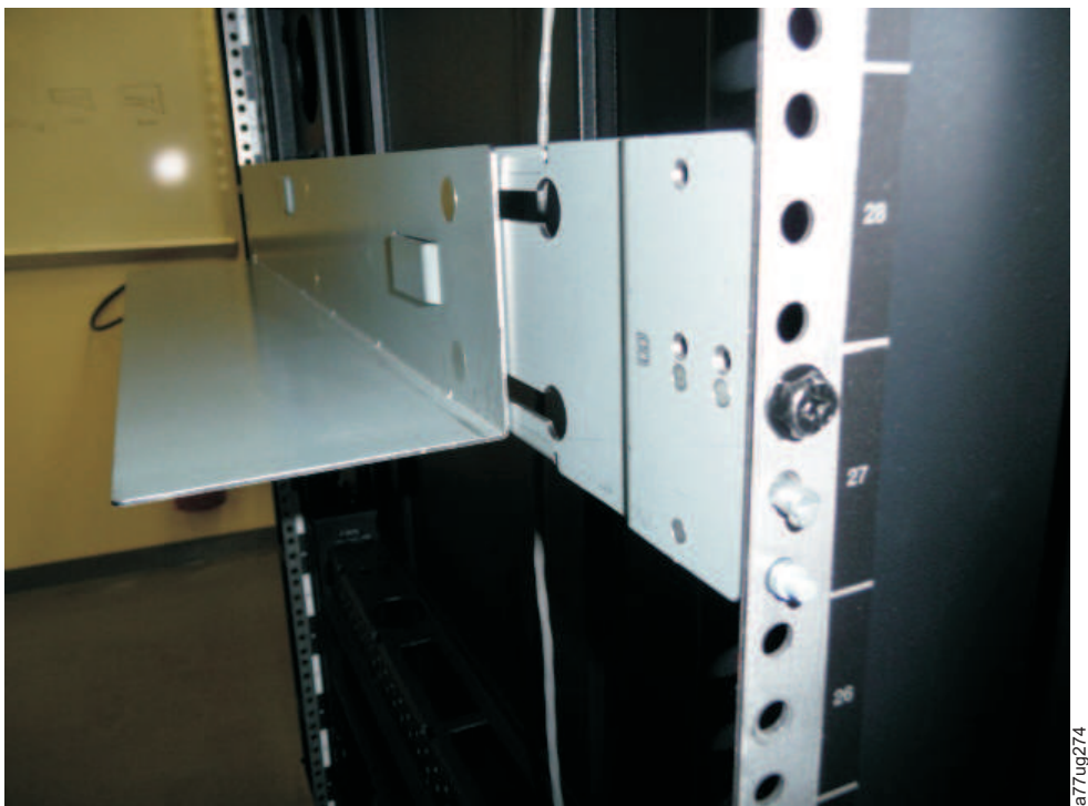
Figure 28. Rear view of Rack Kit B shows a different mounting method
